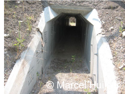
Medium mammal Underpass 1.5-2 m diameter
