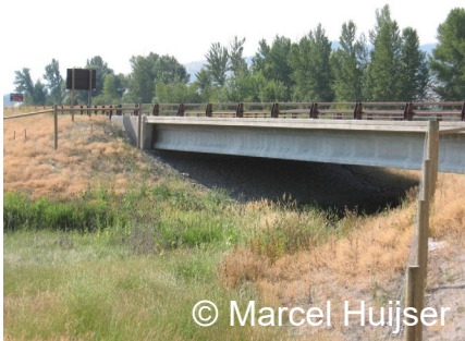
Over span bridge >30 m wide >4-5 m high
