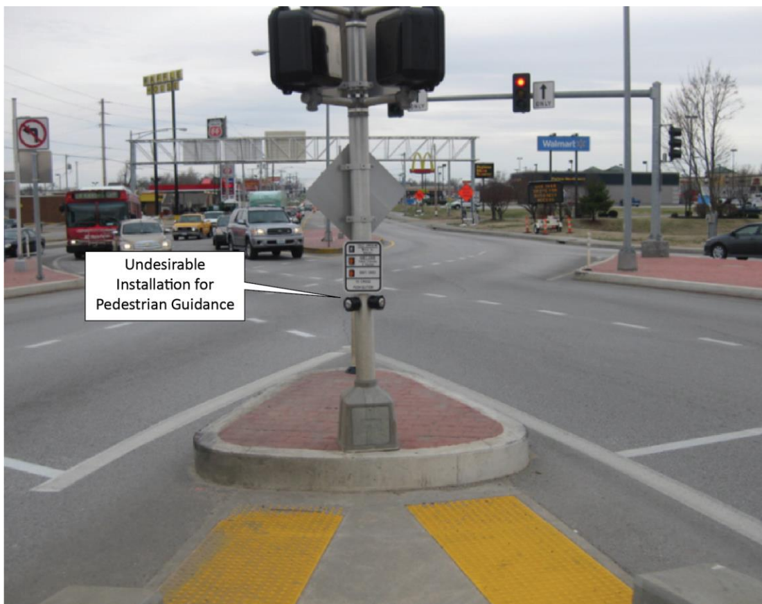
Exhibit 7-12 Undesirable Use of Single Pole with Two Pedestrian Push Buttons, No APS, and Insufficient Separation of the Two Detectable Warning Surfaces
