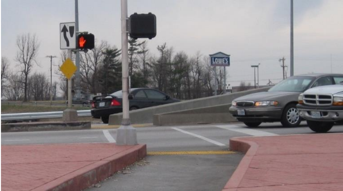
Exhibit 7-14 Pedestrian Signal and Push Button on Outside of Crossover (Pedestrian Facility in Median)
