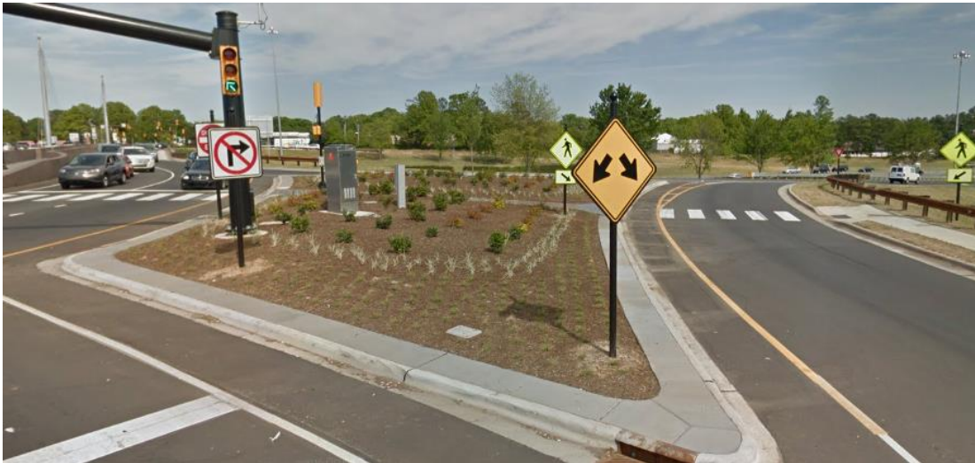
Exhibit 7-2 Signal Cabinet Located in a Landscaped Median with Good Visibility
