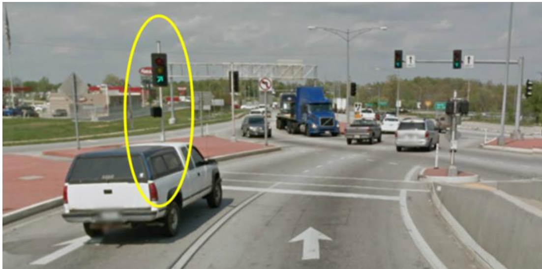
Exhibit 7-9 Supplemental Signal on Left for an Outbound Movement at a DDI
