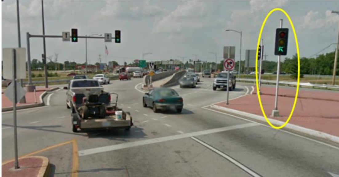
Exhibit 7-8 Supplemental Signal on Right for an Inbound Movement at a DDI
